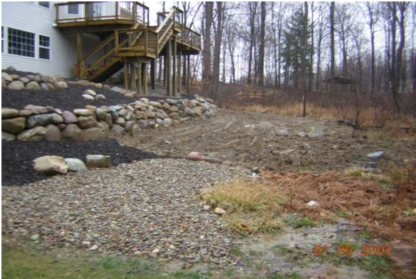
Photo 61: View N along CE on SL 102. New landscaping.
