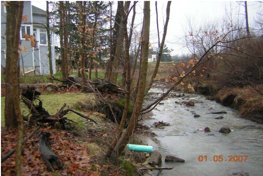
Photo 53: View SW along CE on SL 47 where it crosses the stream.
