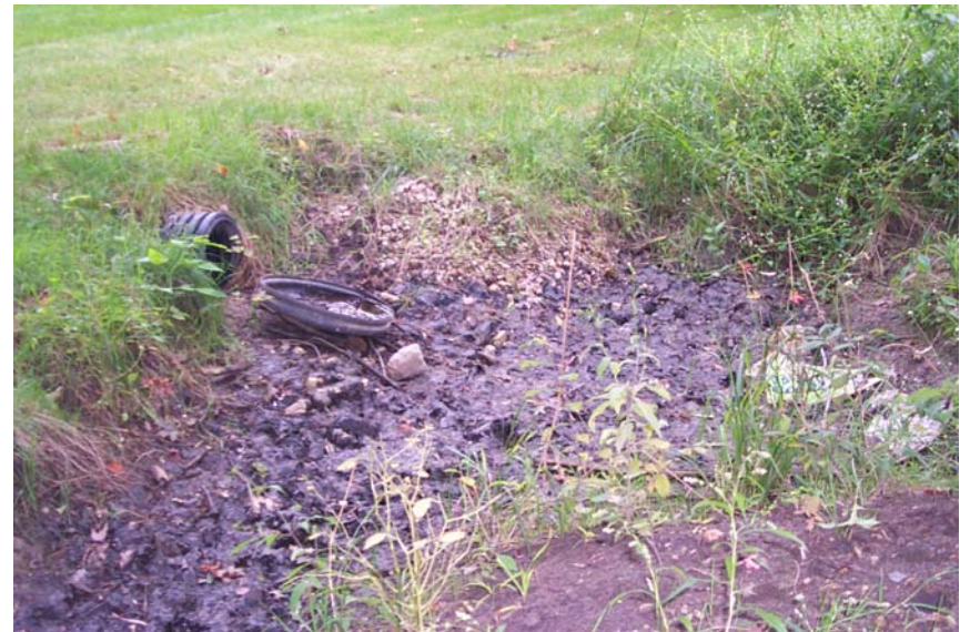
Photo 16: Drainage from SL 22 into drainage basin in CE.
