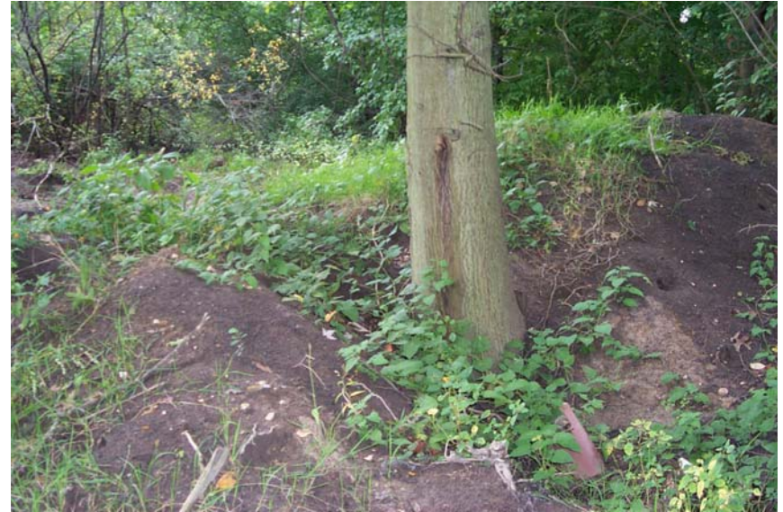
Photo 18: Fill from dug out pond along its edge in CE, off SL 22.
